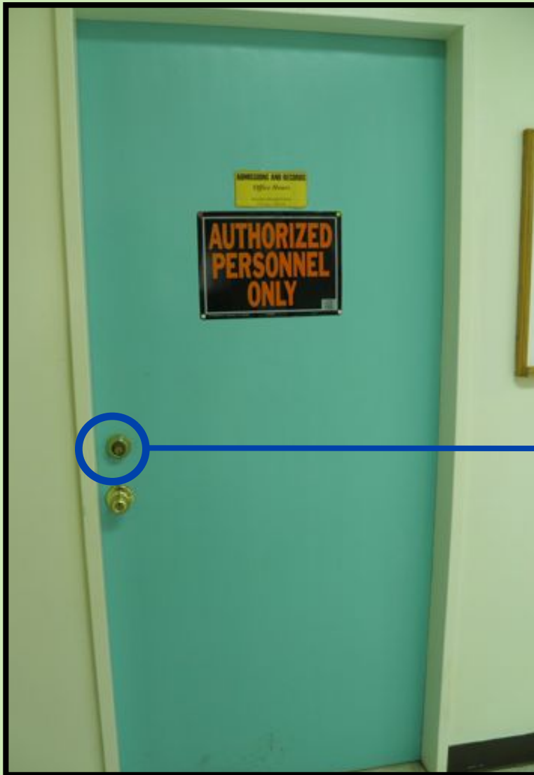
Figure 3.0. The Office's main entrance door now fitted with an additional locking mechanism (dead bolt).
